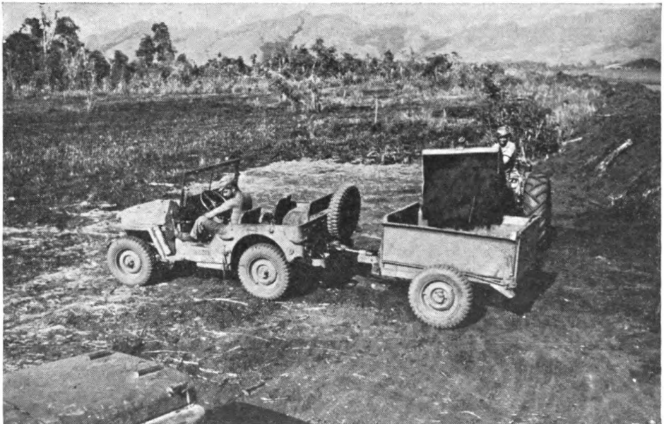
Figure 7. Loading ½-ton dump trailer with shovel loader on rubber-tired tractor.
